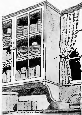
Built-in cupboards save time and labor
