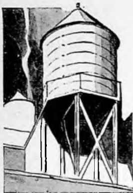
Tanks give adequate pressure and supply
