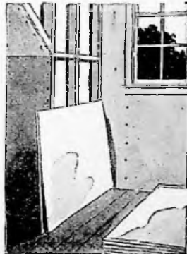
Wall board, paint, transform the basement
