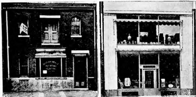
A clever architect plus a progressive owner equals a new store front and more business
